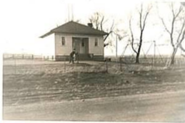
Old Lace School House at the corner of Cass and 75 th Street which also housed the first City Hall and Police Department (all that in this one small place!)
