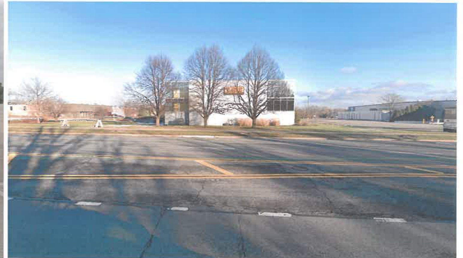
View from West Side of Building
