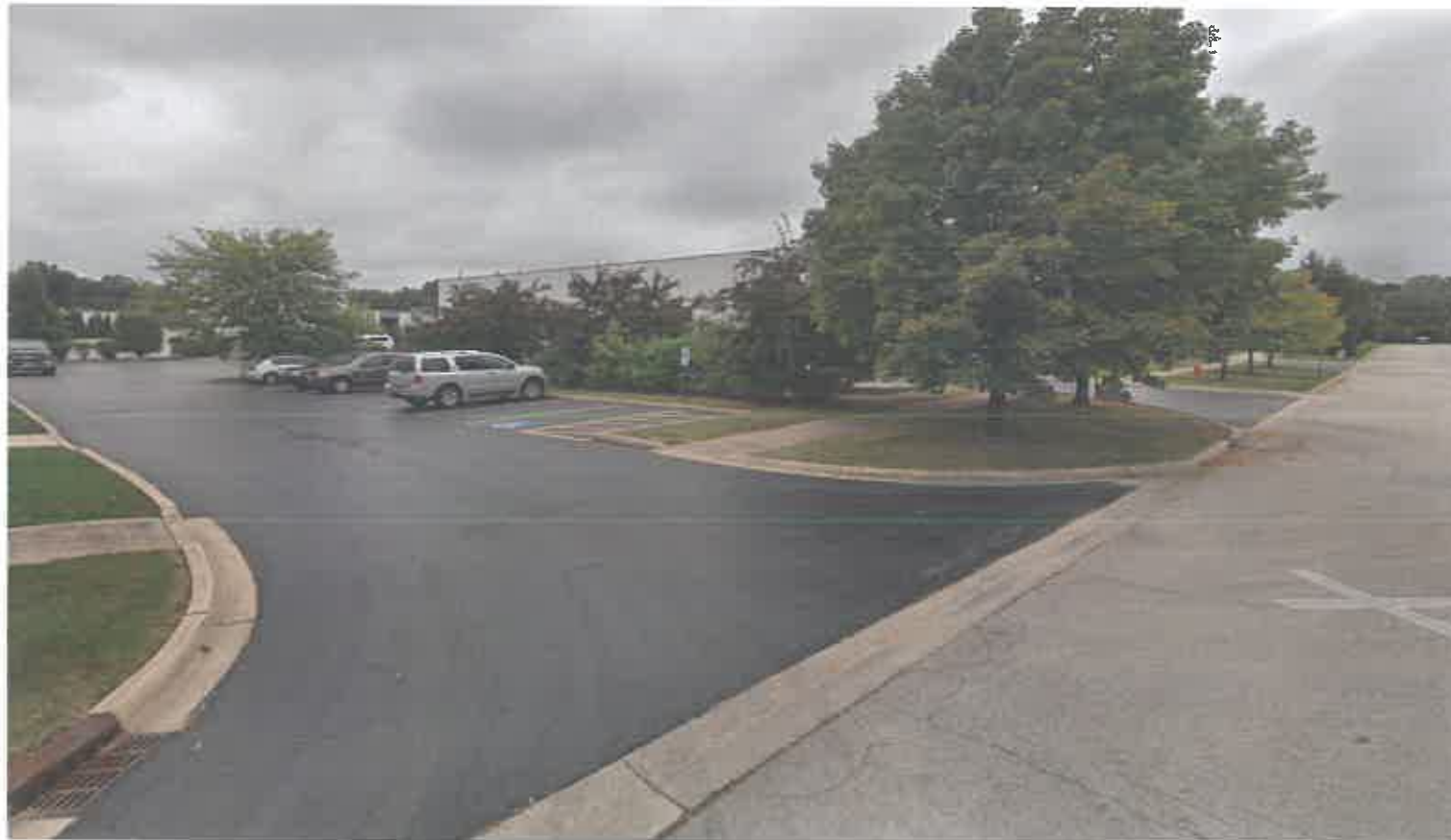
View from East Side of Building
