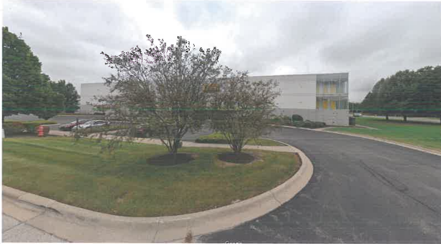
View from North Side of Building
