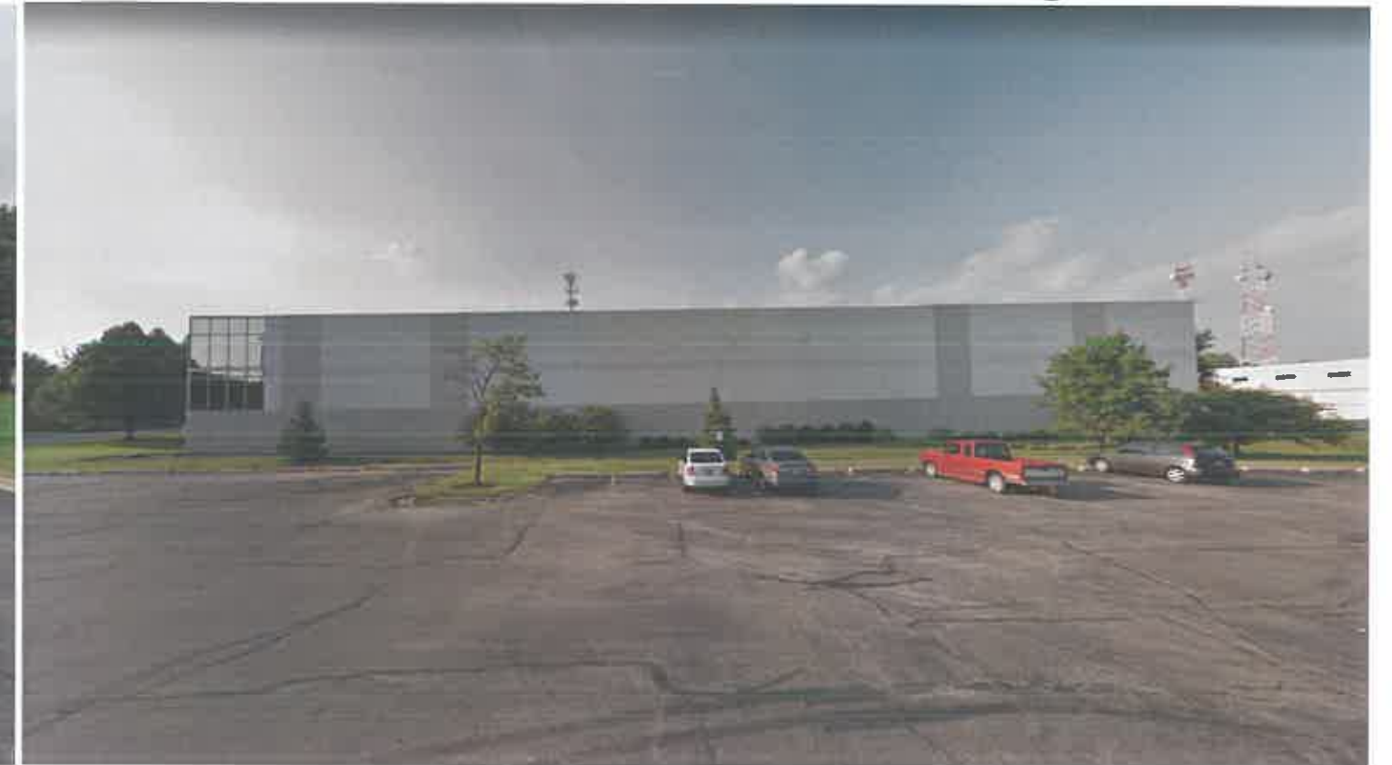
View from South Side of Building
