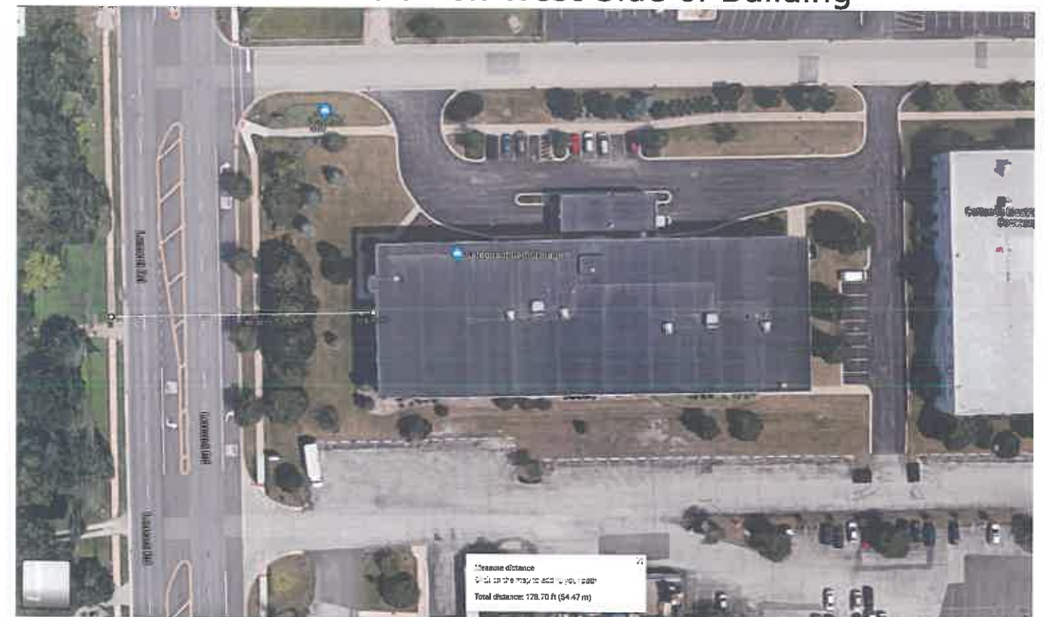
Dimension on West Side of Building
