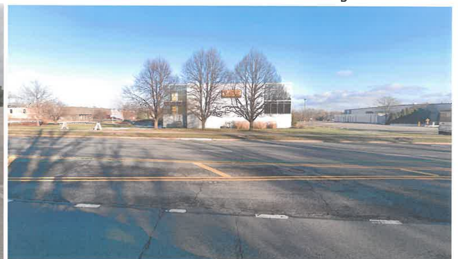
View from West Side of Building
