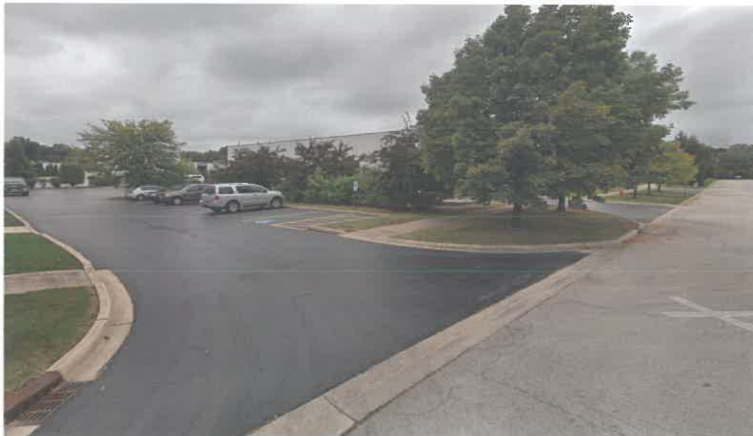
View from East Side of Building
